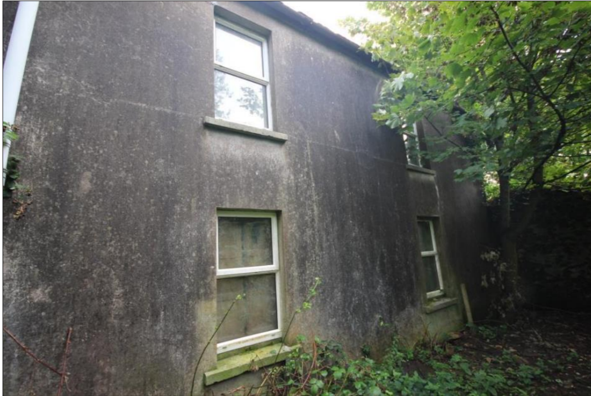
Plate 35: Front elevation with cement render
