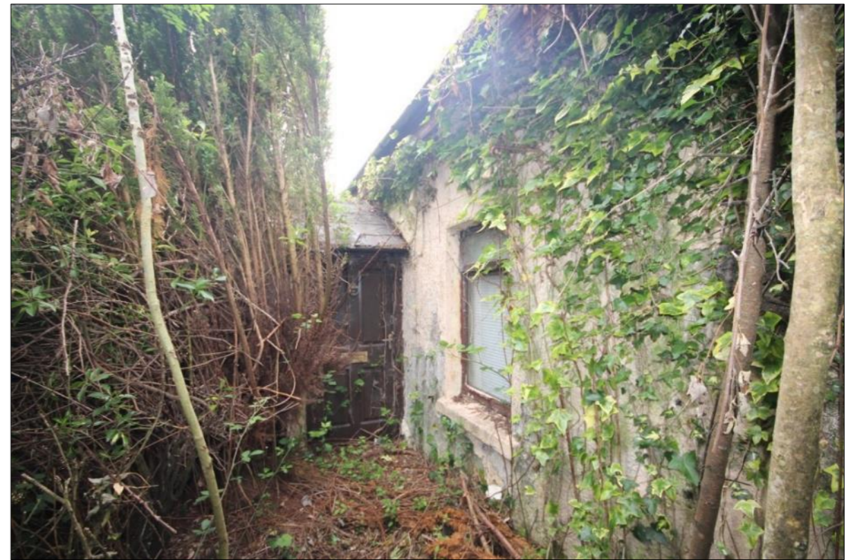
Plate 15: Southern elevation and porch
