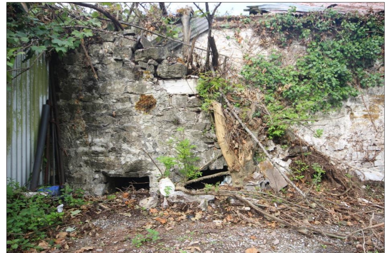
Plate 59: Steps and opening in eastern elevation of Building C- Western outbuilding
