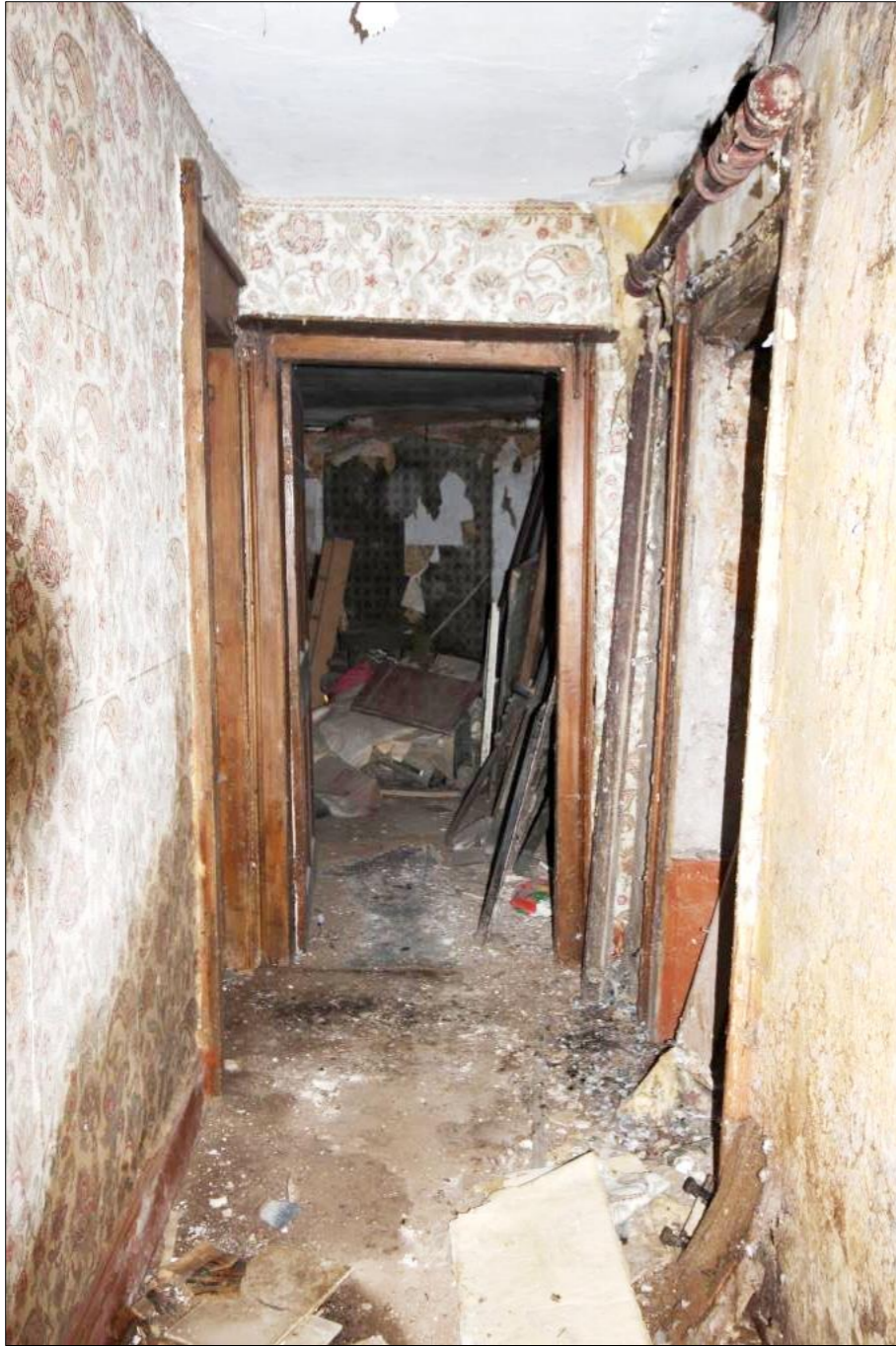
Plate 41: Ground floor hall GF04
