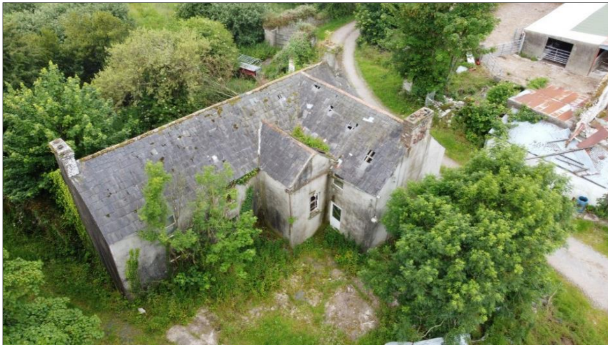
Plate 26: View of Maglin House looking southwest showing rear (northern) elevation
