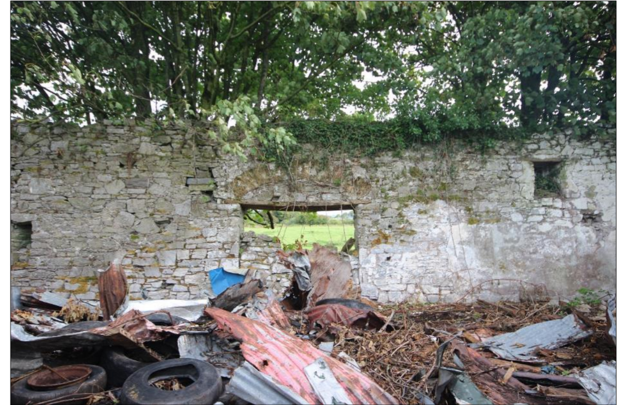
Plate 66: Interior of northern range looking north
