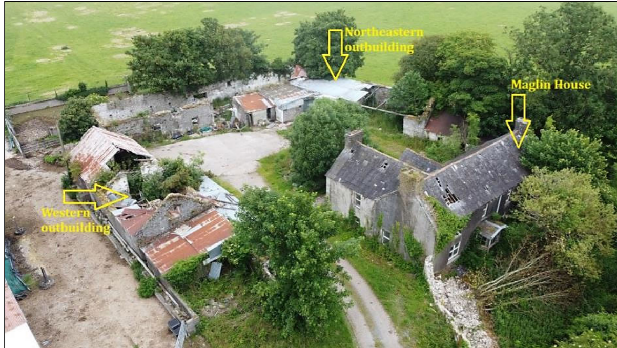
Plate 56: General view of farm complex
