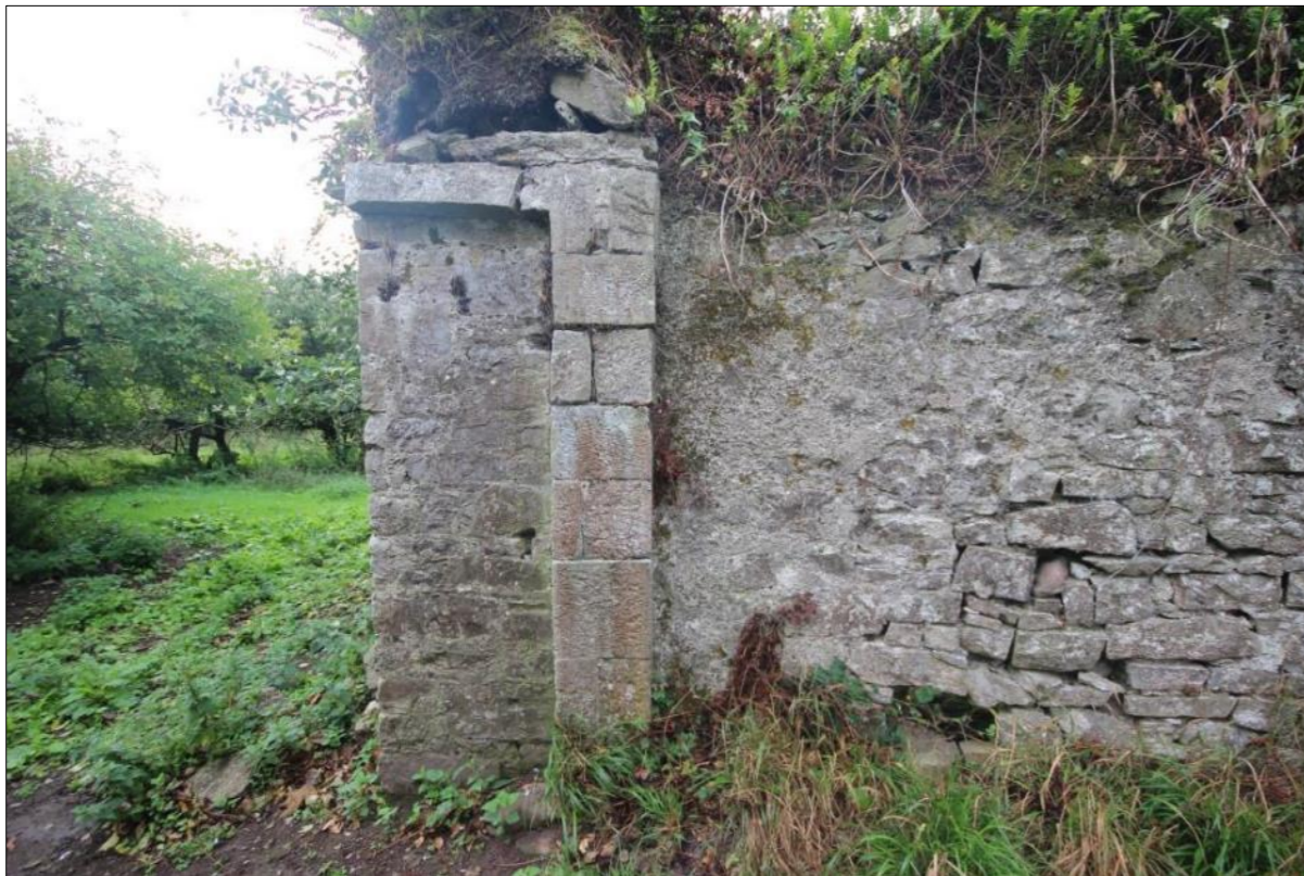
Plate 73: Cut-stone pier to entrance to Building E-Walled orchard
