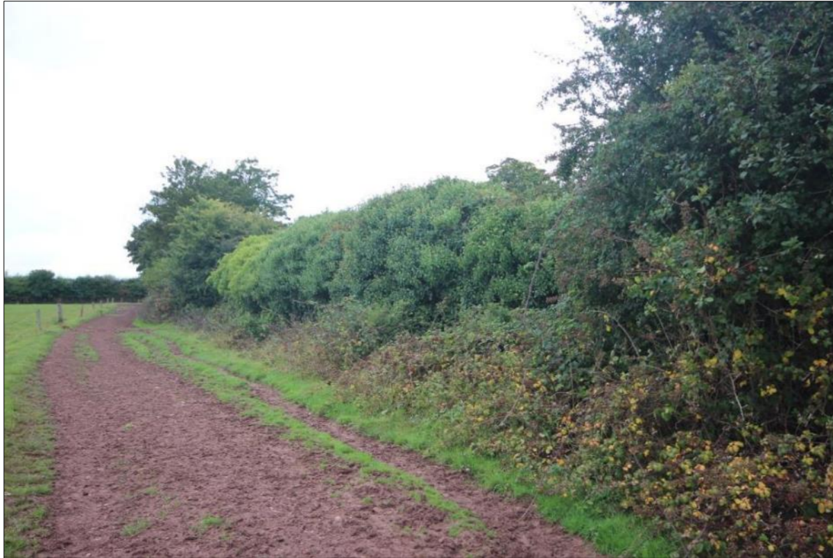
Plate 76: Overgrown southern wall of Building E-Walled orchard
