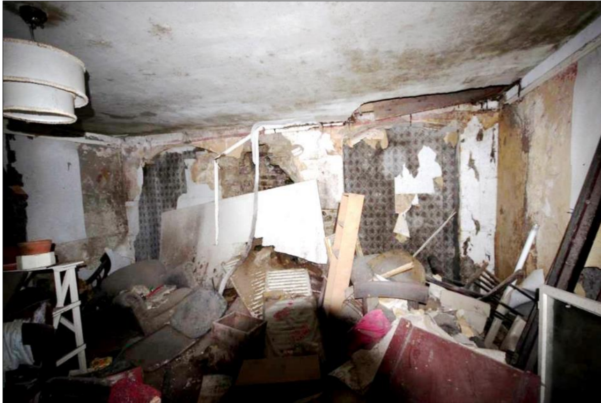
Plate 43: Ground floor room GF06
