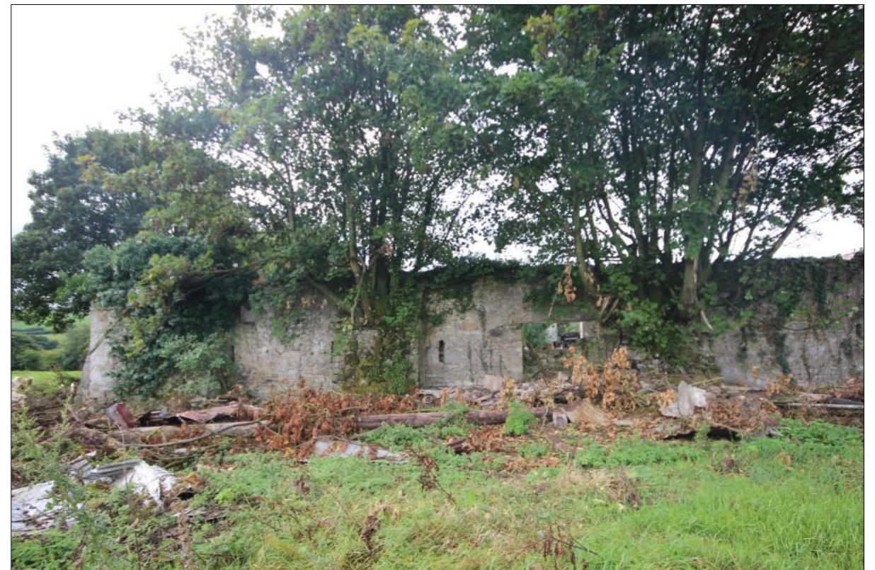
Plate 63: Northern elevation of northern range
