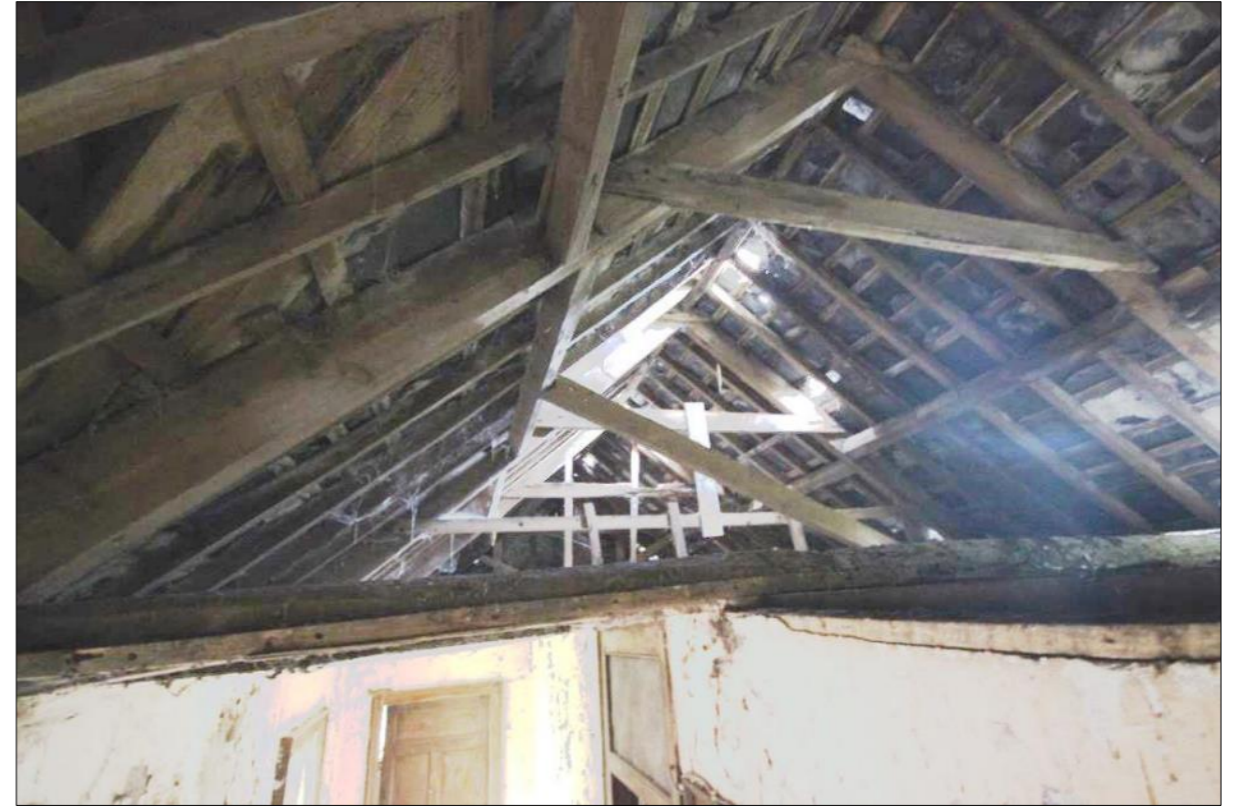
Plate 55: Roof truss detail
