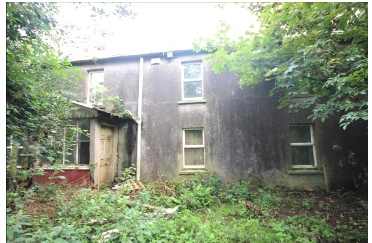
Plate 28: Front (southern) elevation of Maglin House
