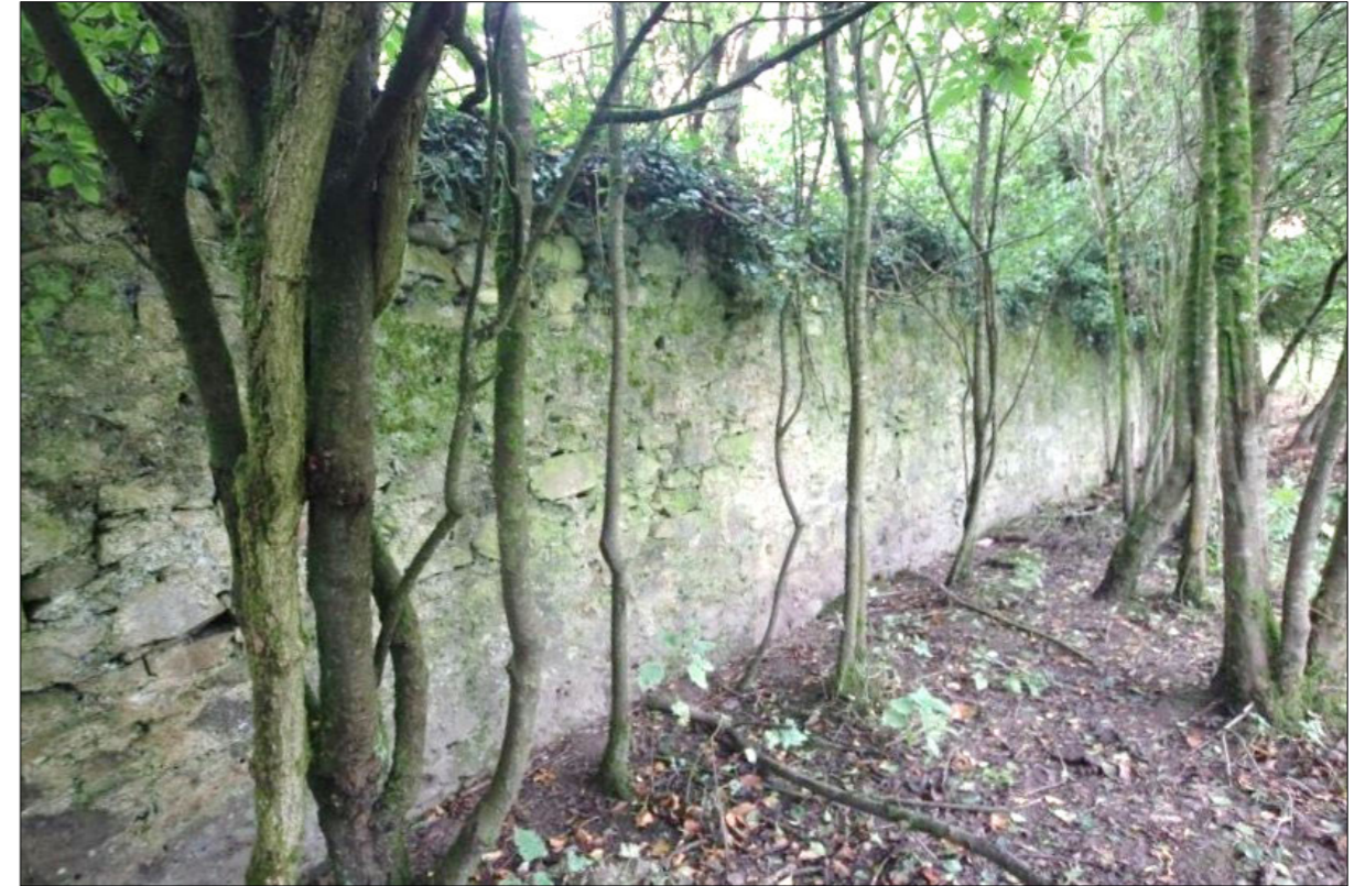
Plate 82: Internal elevation of southern wall of Walled Orchard
