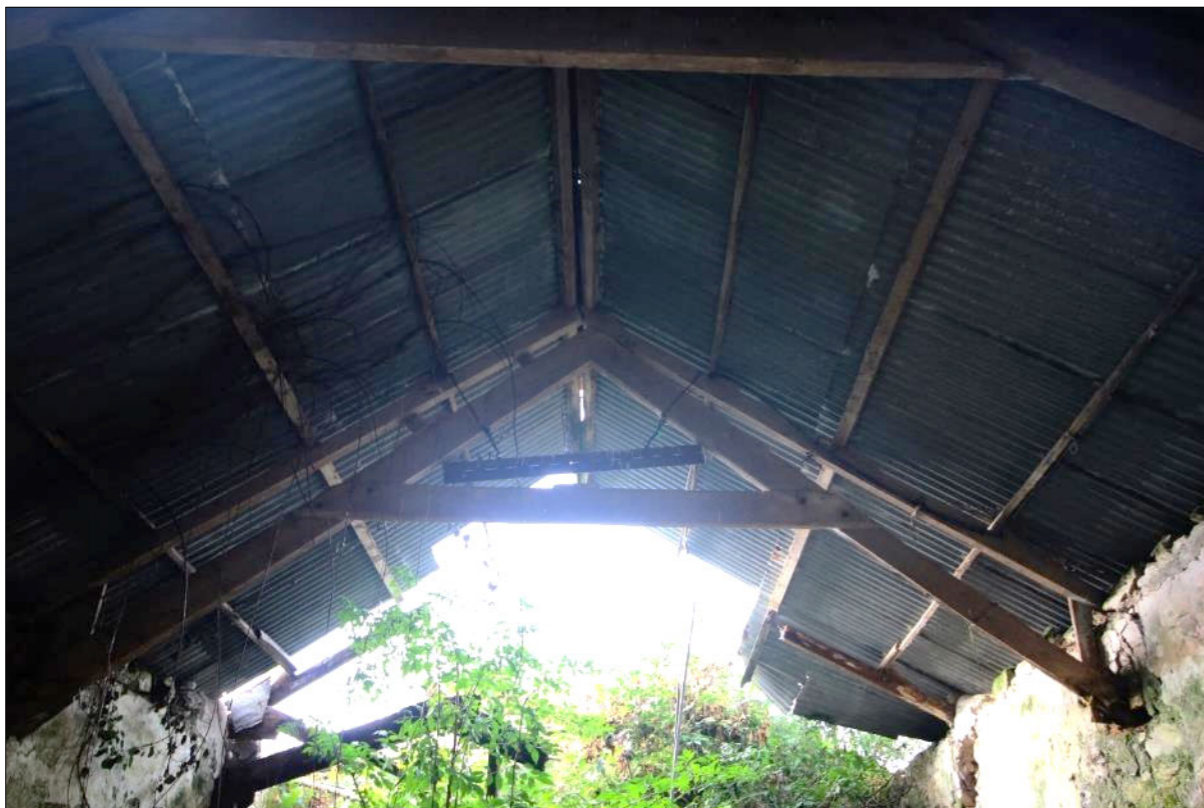
Plate 61: A-framed truss to Building C-Western outbuilding
