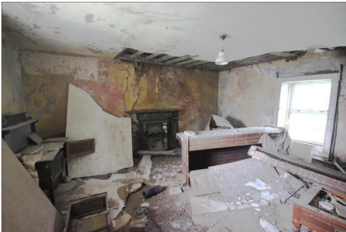
Plate 51: First floor room FF02
