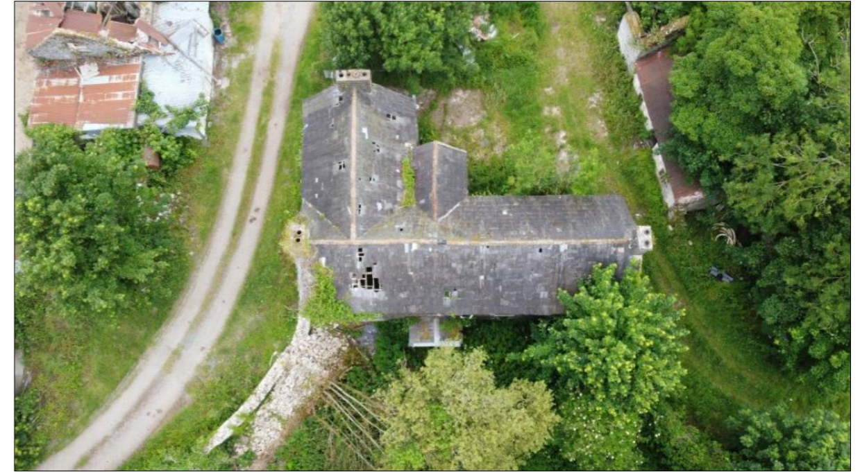
Plate 27: View of roof of Maglin House
