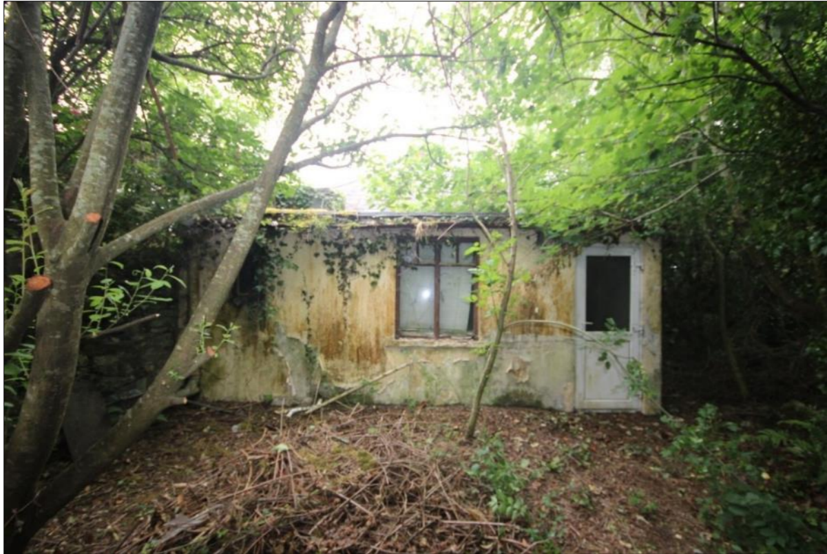
Plate 16: Modern flat-roofed extension to eastern wall
