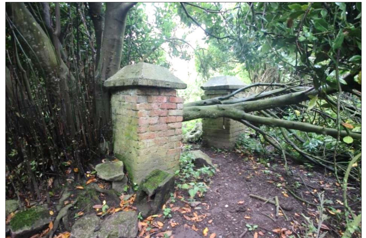
Plate 79: Brick gate piers between Wadded Orchard and Maglin House
