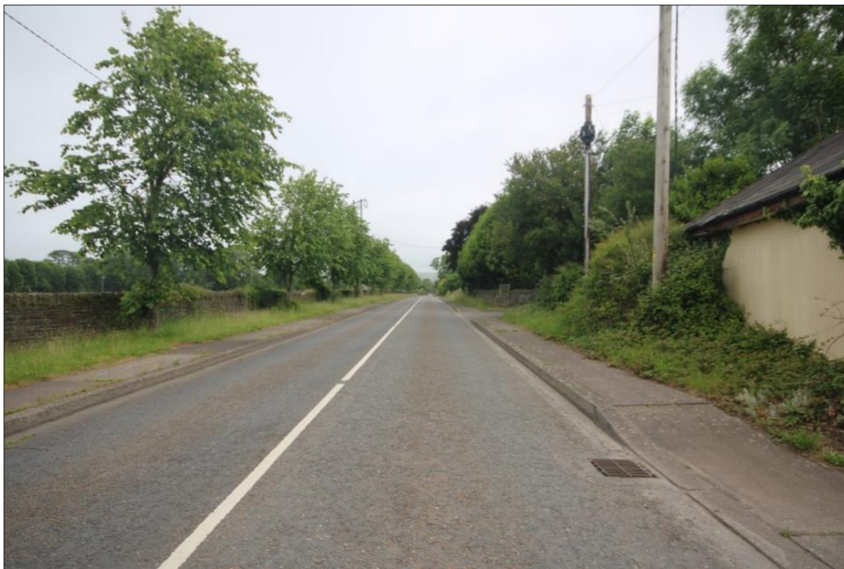
Plate 6: General view along western boundary of subject site on Maglin Road looking north
