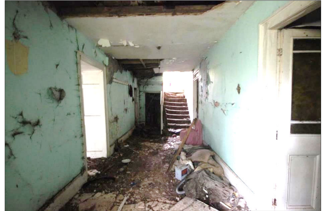
Plate 37: Ground floor entrance hallway GF01 looking to staircase
