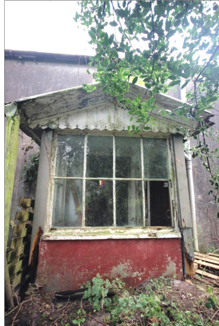
Plate 34: Porch to front elevation
