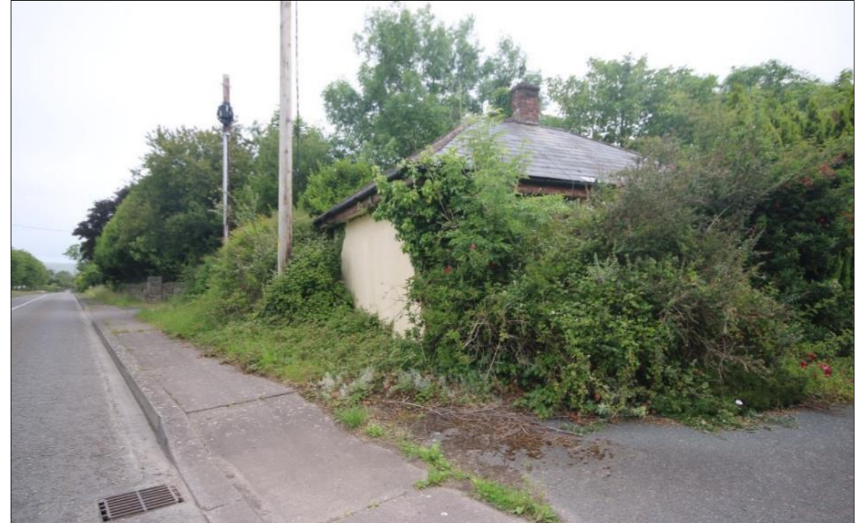
Plate 14: Western elevation to roadside
