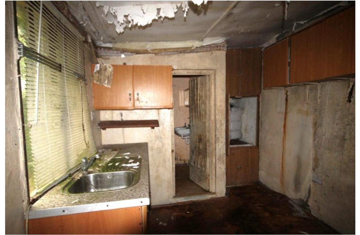
Plate 24: Kitchen and WC in modern extension GF04
