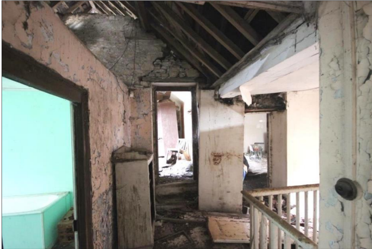
Plate 50: First-floor landing FF01 looking to FF05 and FF06
