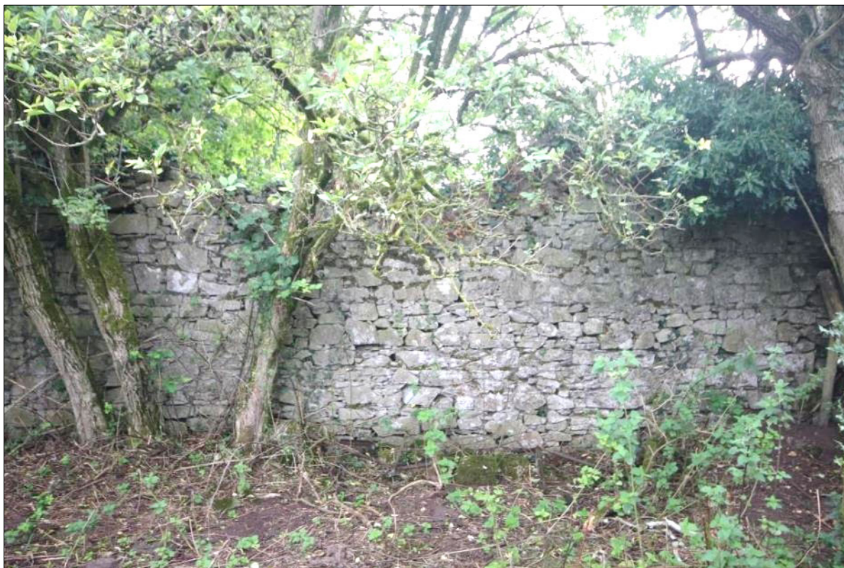
Plate 81: Internal elevation of eastern wall of Walled Orchard
