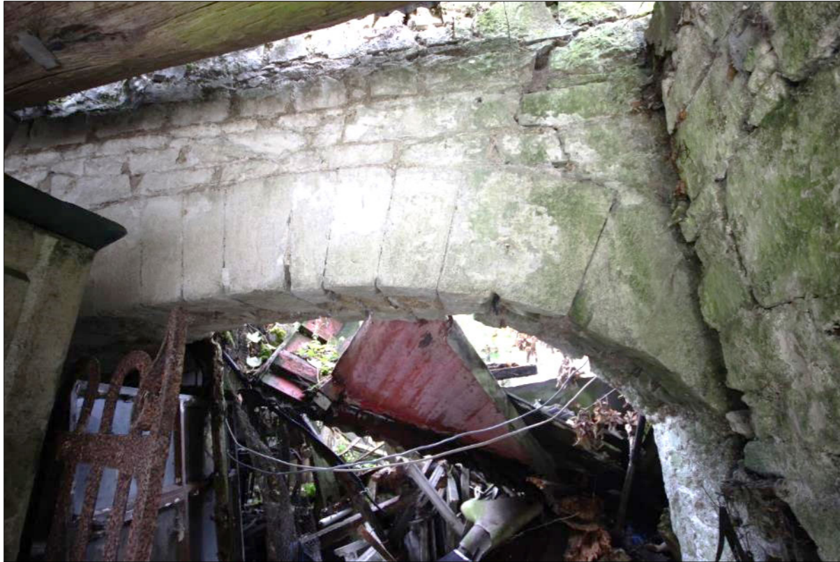
Plate 60: Archway in Building C-Western outbuilding
