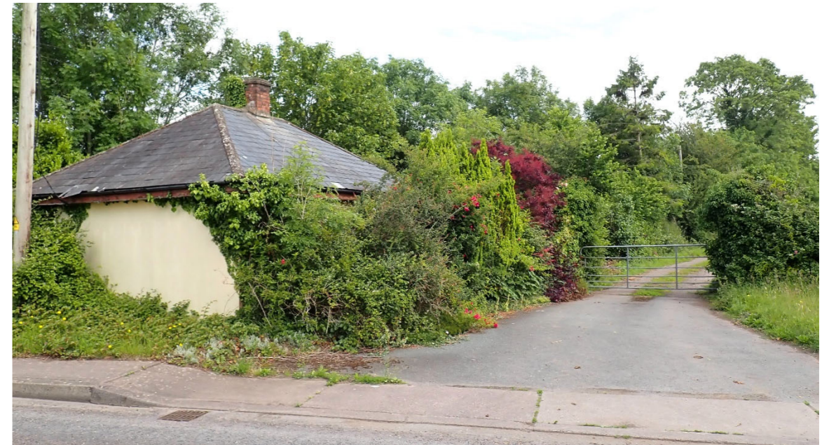
Photo 9.3.1: View East of site access and old gate lodge on Maglin Rd. on western boundary.
