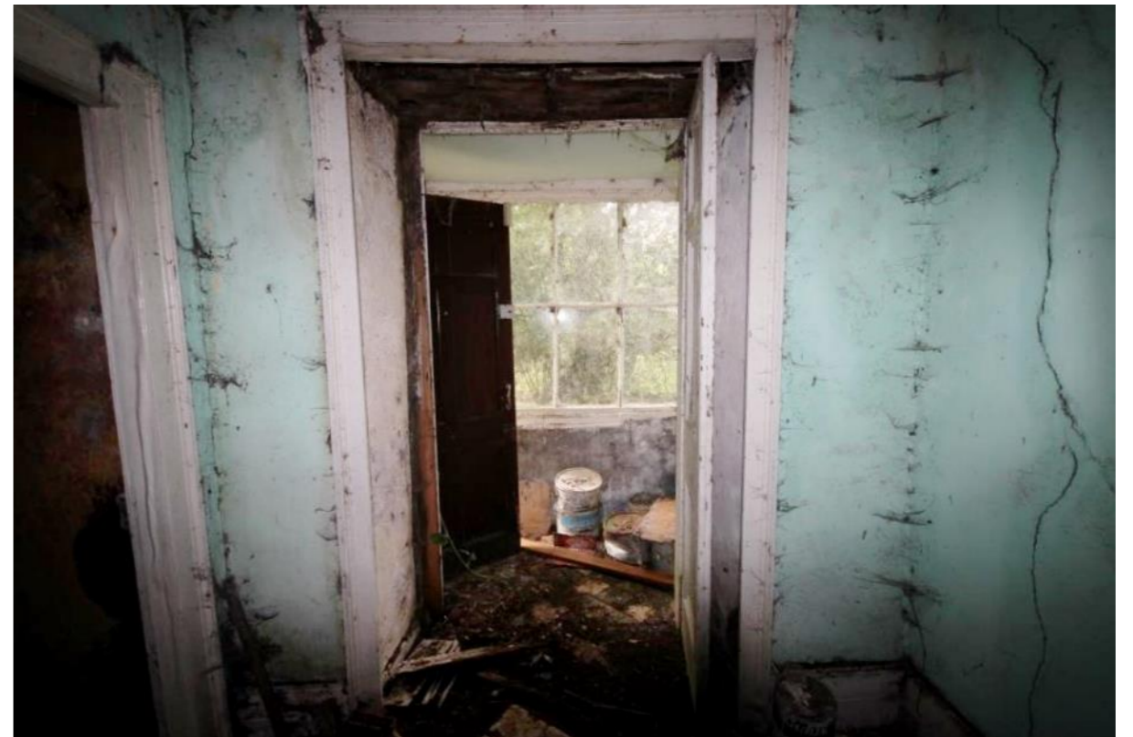
Plate 38: Ground floor entrance hallway GF01 looking to porch
