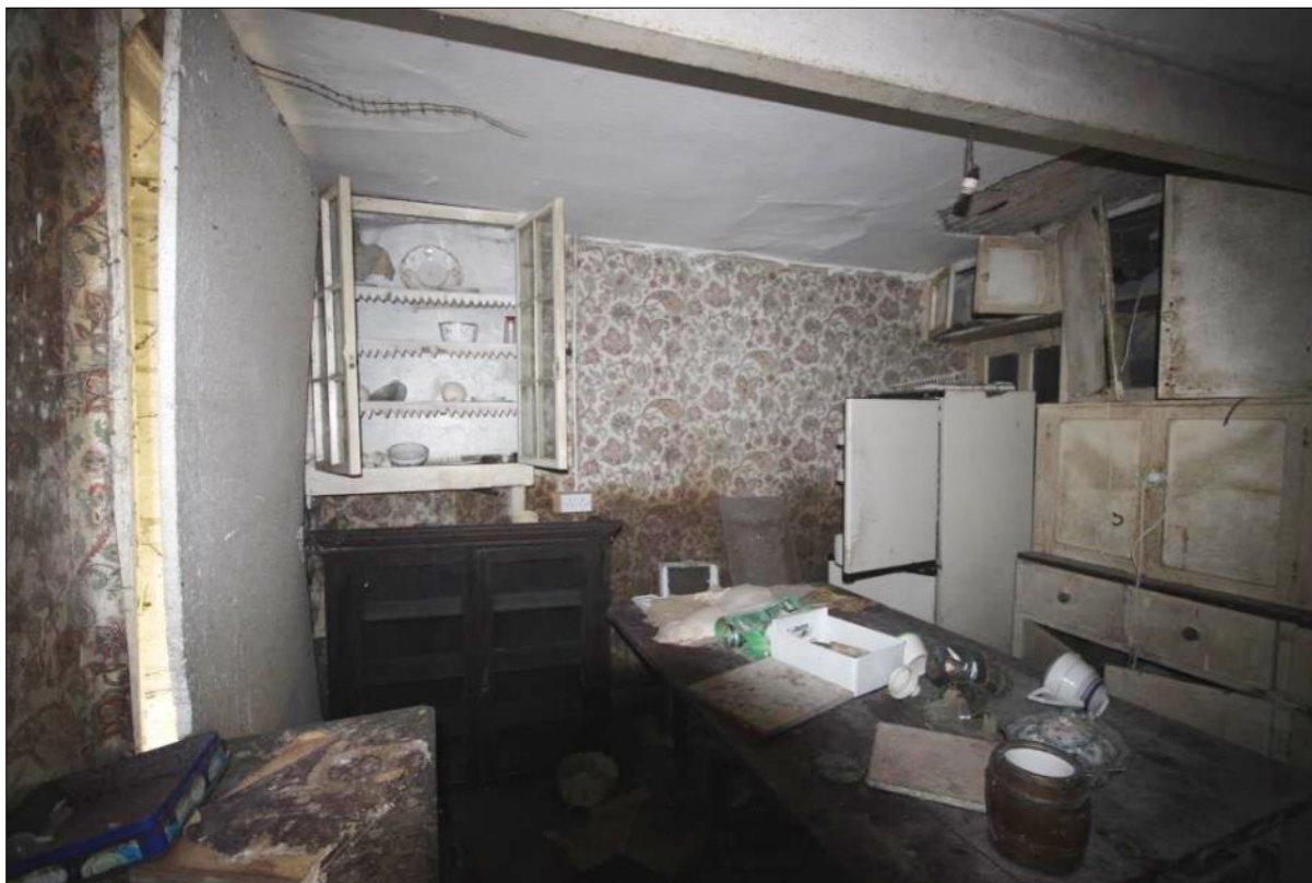
Plate 44: Ground floor room GF05
