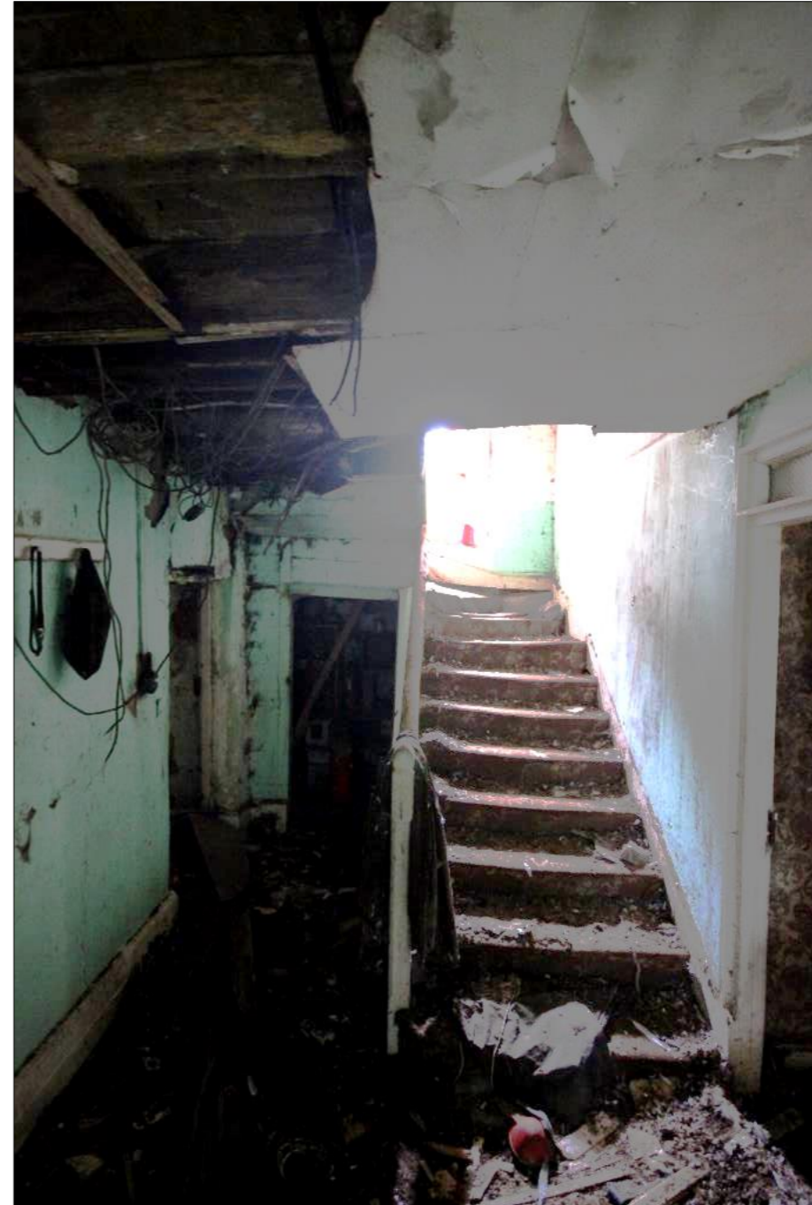
Plate 45: Staircase in hallway
