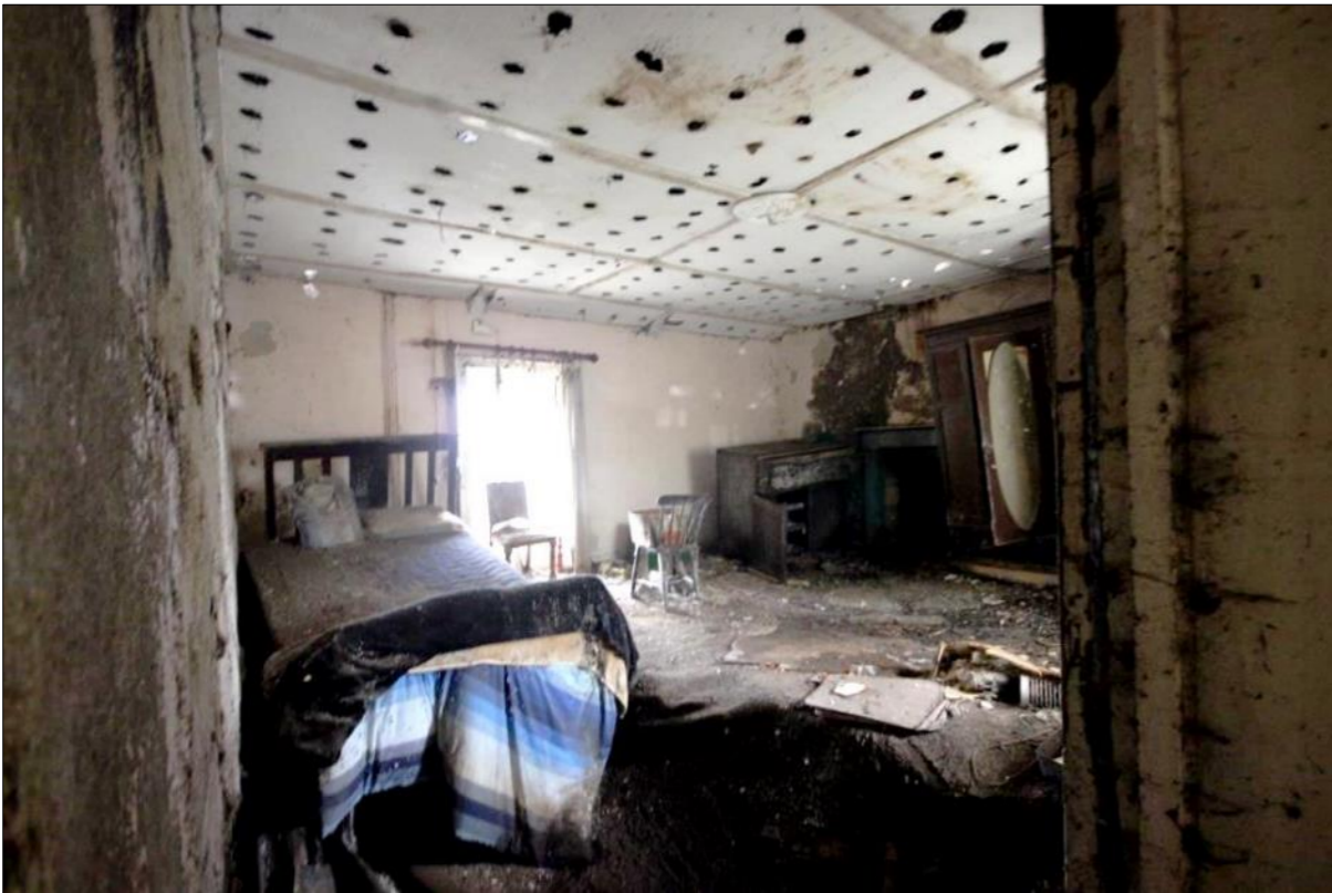
Plate 54: First-floor bedroom in return FF06
