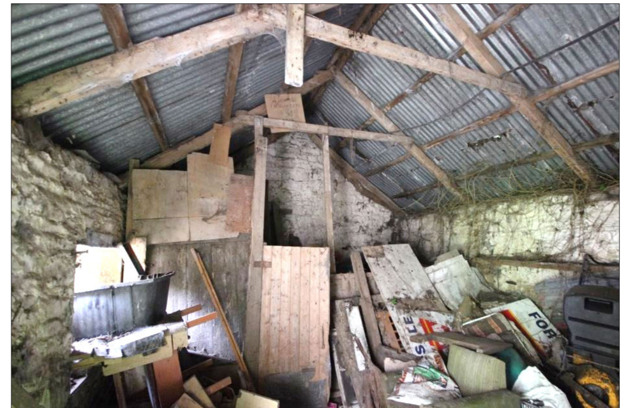
Plate 71: Interior of workshop
