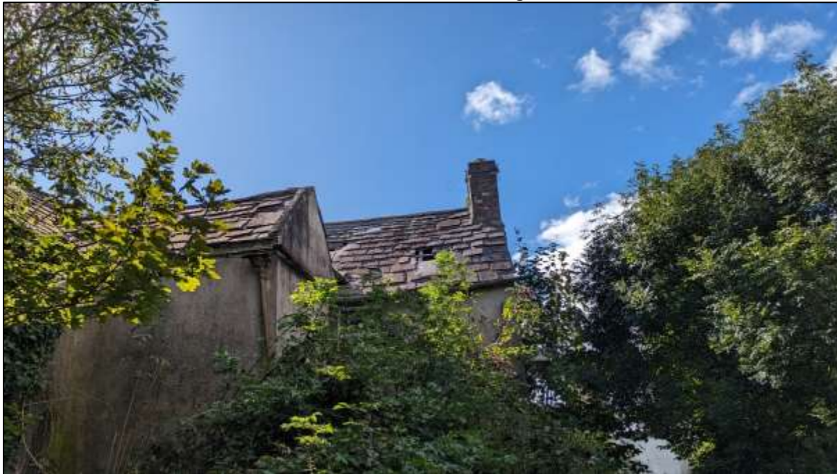
Plate 3-1: Building onsite with features suitable for roosting bats
