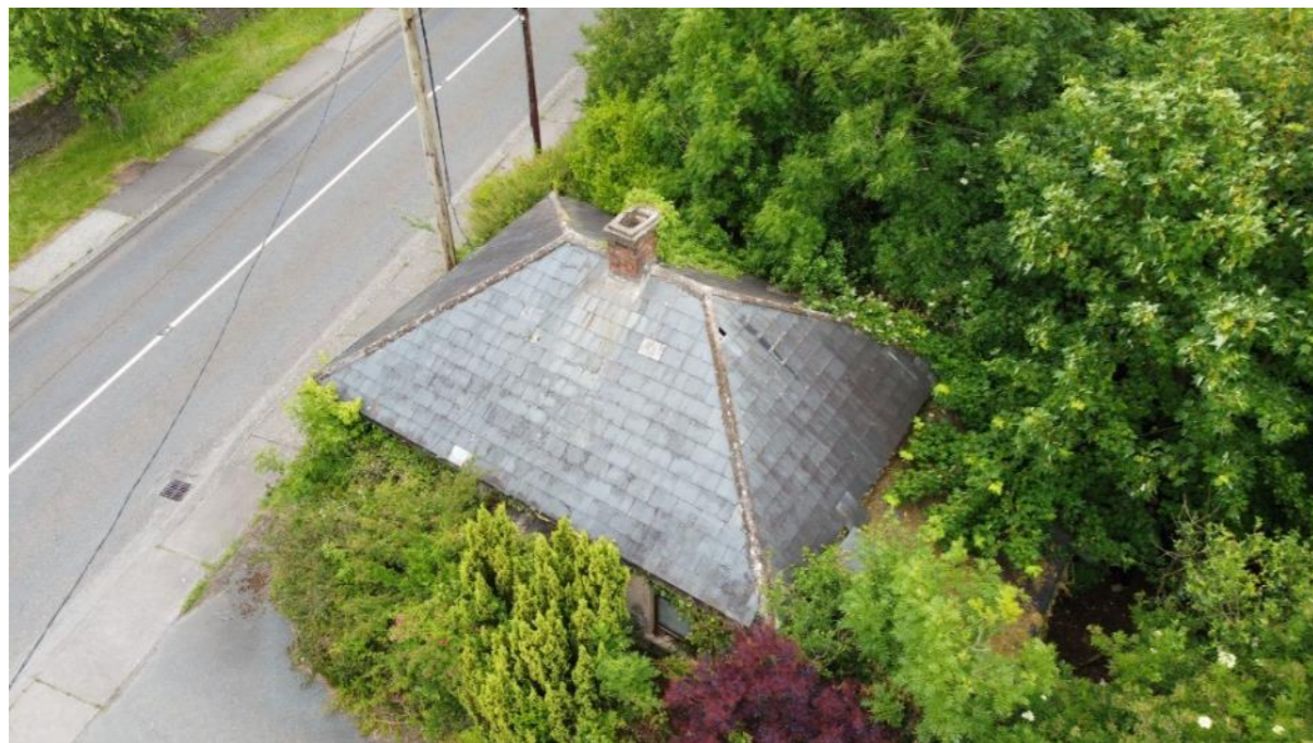
Plate 17: Roof of gate lodge
