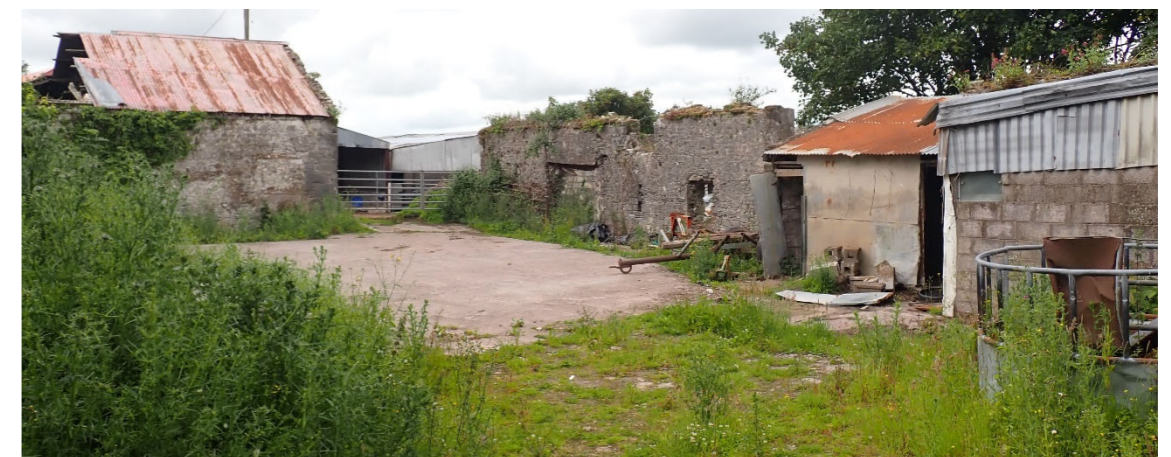
Photo 9.3.26: Old out houses and sheds in farm yard area on north side of Maglin House.
