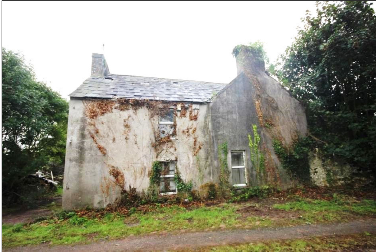
Plate 29: Western elevation of Building B-Maglin House
