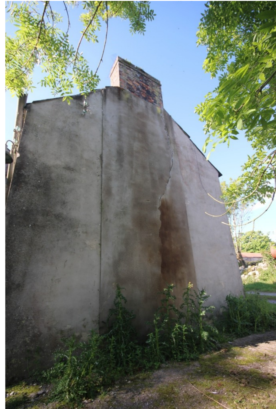
Plate 31: Eastern elevation of Building B-Maglin
