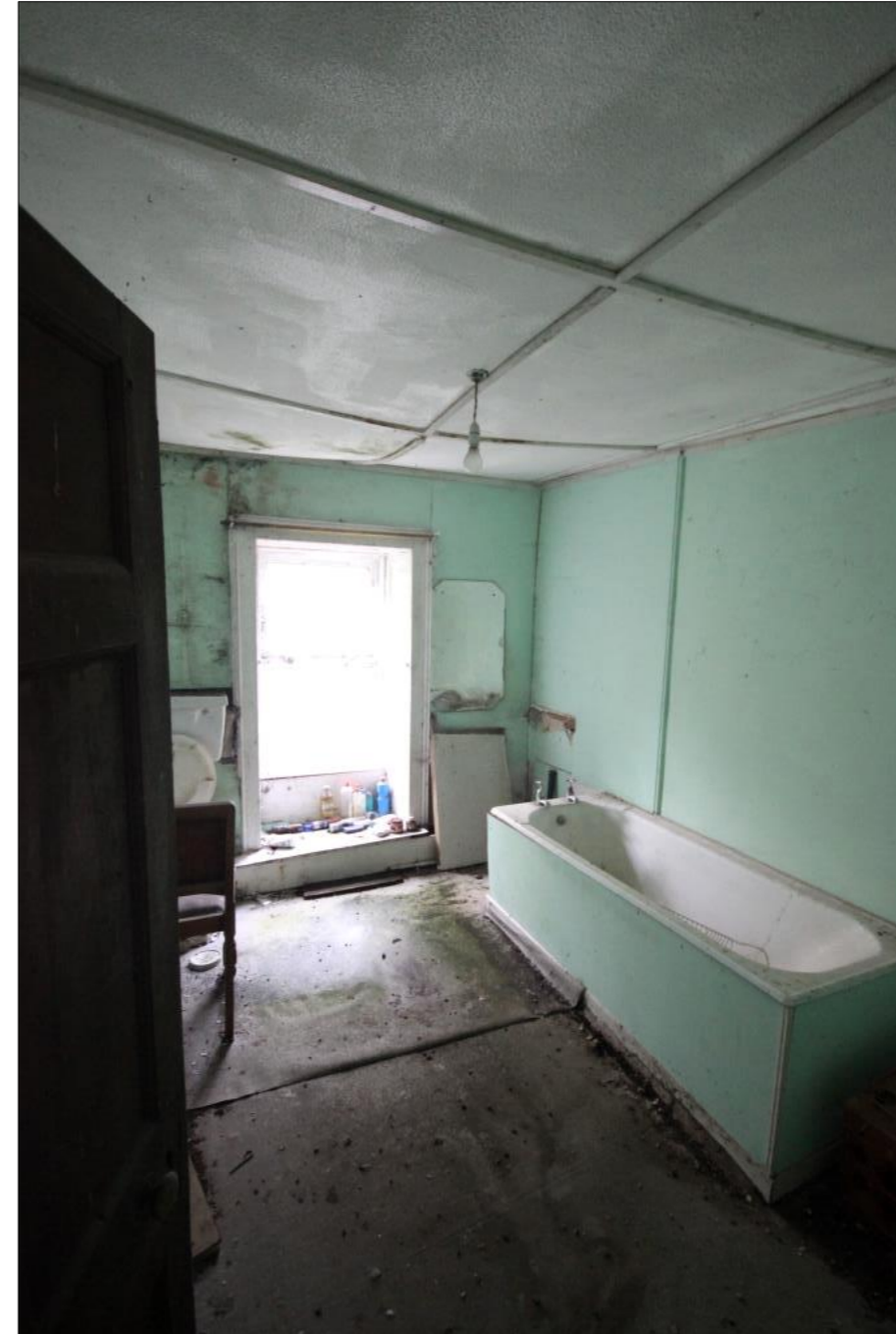
Plate 52: First-floor bathroom FF04
