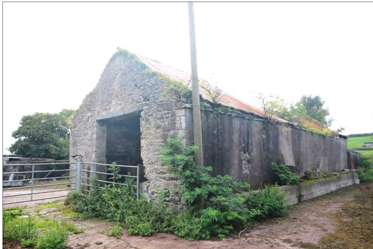
Plate 57: Northern and western elevation of Building C-Western outbuilding
