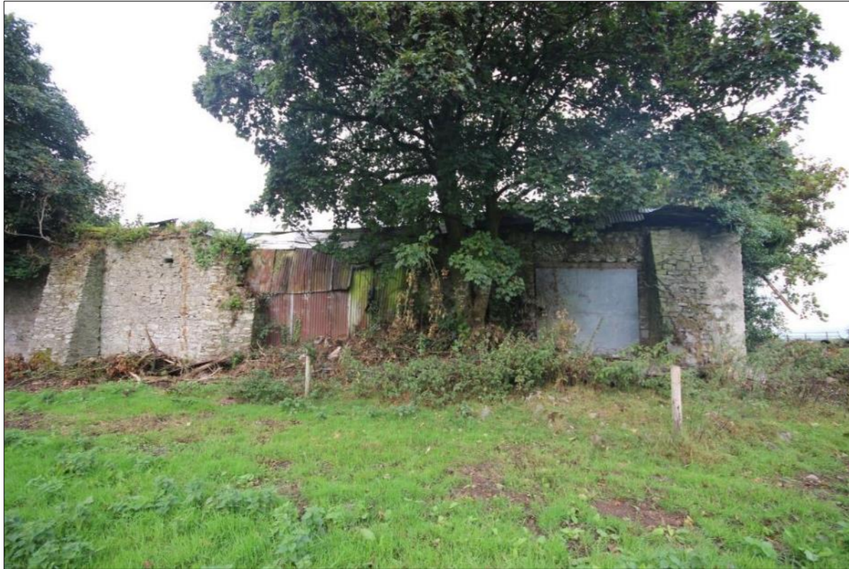
Plate 64: Eastern elevation of northern range
