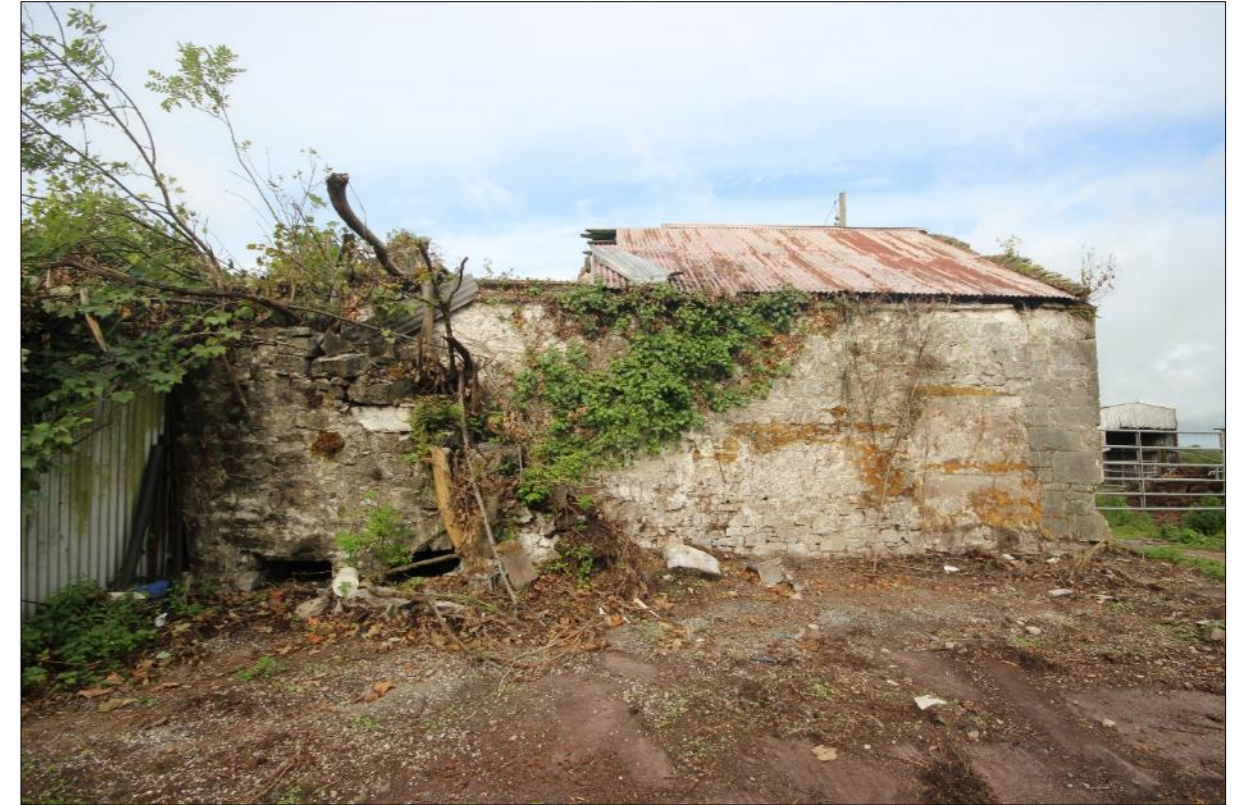
Plate 58: Eastern elevation of Building C-Western outbuilding
