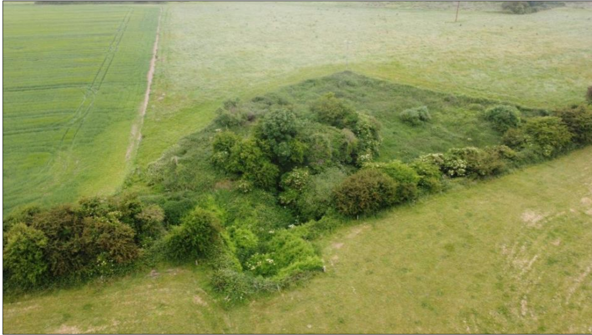
Plate 5: General view of overgrown lime kiln to north of subject site
