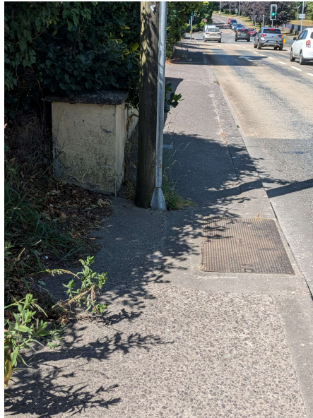
Figure 5.3 Pinch point along footpath
