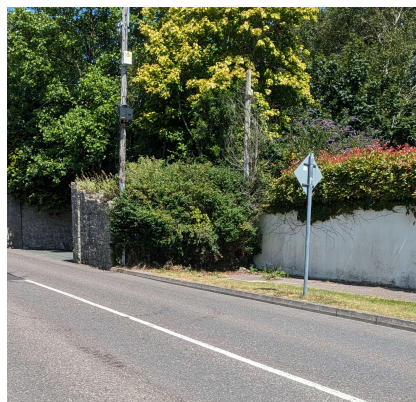
Figure 7.2 Abrupt end to footpath
