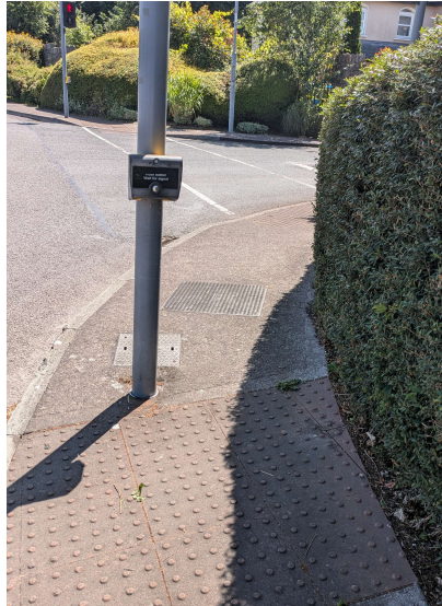
Figure 5.5 Pinch point along footpath
